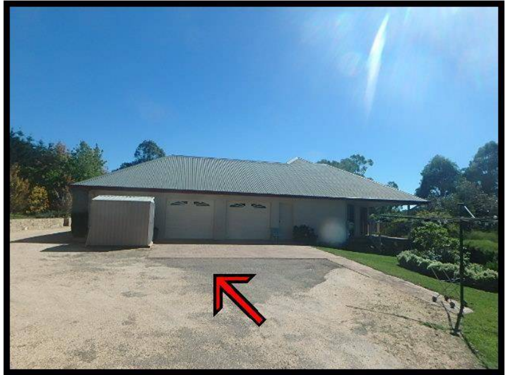
The gravel driveway stands in fair condition.
