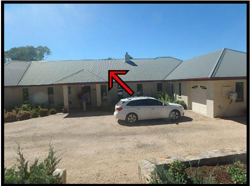
The overall condition of the roof coverings is good.
